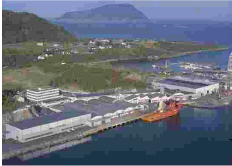
RRM – Brattvaag CoE (Deck machinery)
